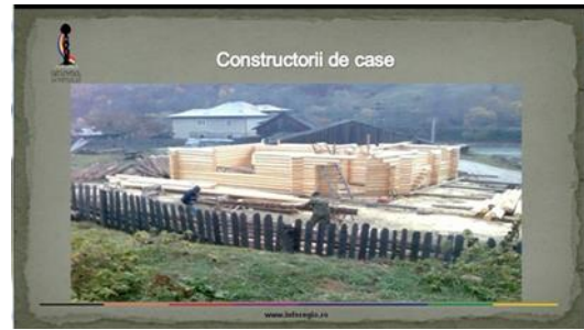
Plate 4 ( SLH , wooden house being built)
